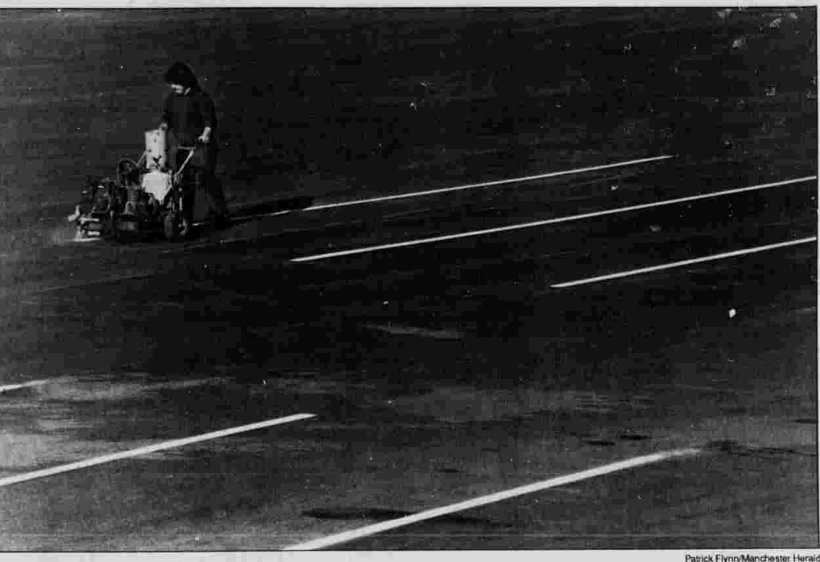
A LOT OF WORK — Lance Raybigne lines parking spaces this week in a lot near the Pavilions at Buckland Hills.
